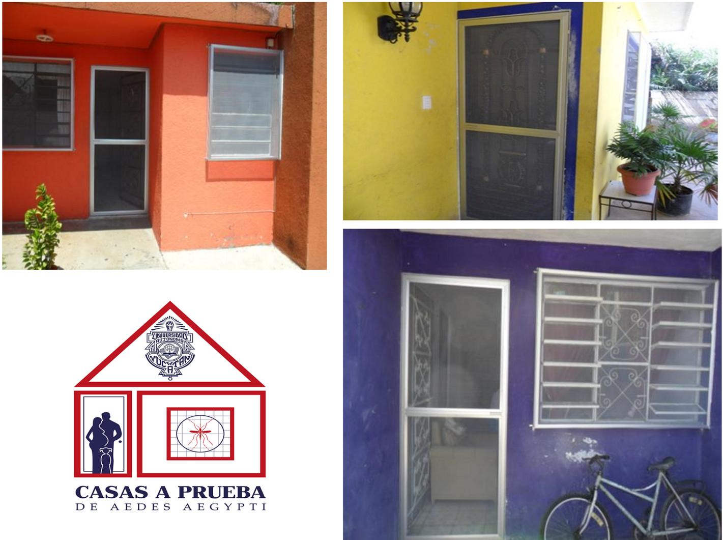
**Fig 2. House screening with insecticide-treated netting.** Photographs show housing improvement with insecticide-treated screens mounted on aluminium frames and fixed to external doors and windows of treated houses in Merida, Mexico.
